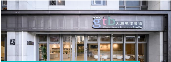
Energy Management & Environment Monitoring System at GTB Plaza A7
